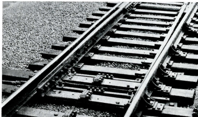
Conventional type switch point
