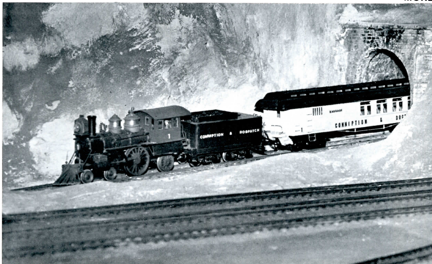
The prototype for this cute little "bicycle" 4-2-2, scratchbuilt by Mac McArthur, is Baldwin Locomotive Works No. 5000. The motor is in the tender. Mac's scratchbuilt combine also contains a motor and his own custom gear train. The combine's sides are formed from photoengraved zinc.
