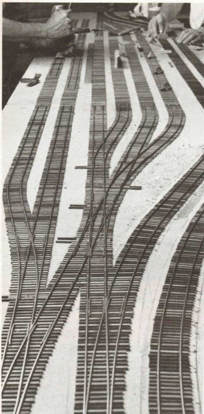
Here's the gang laying track. Looks great!
