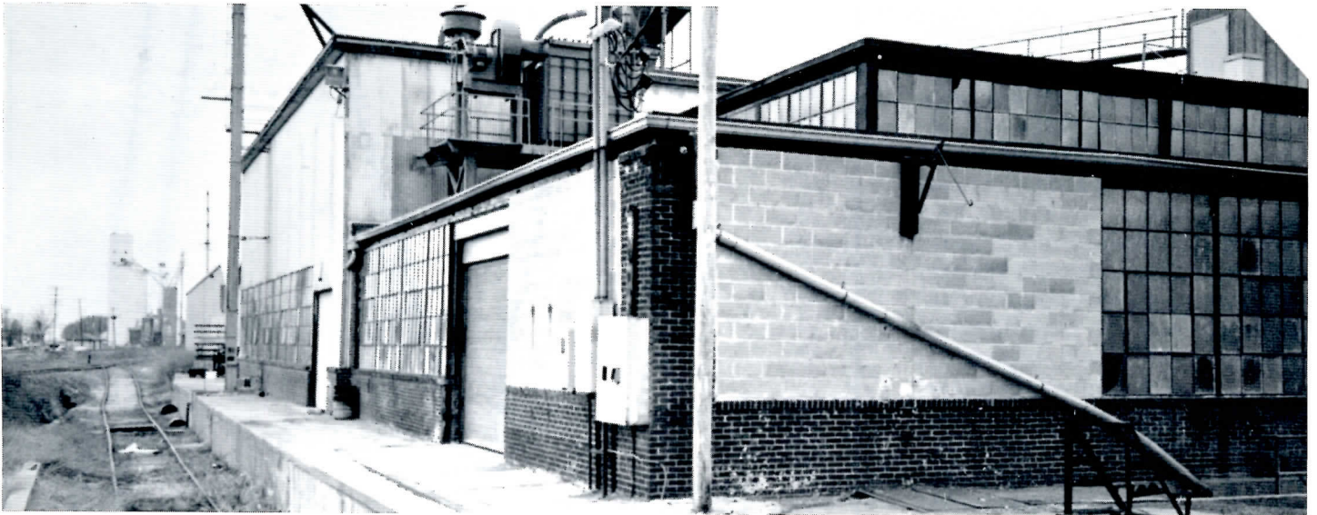
A view from the North showing pocket for hopper car. Note the machinery on top of low portion of building.
