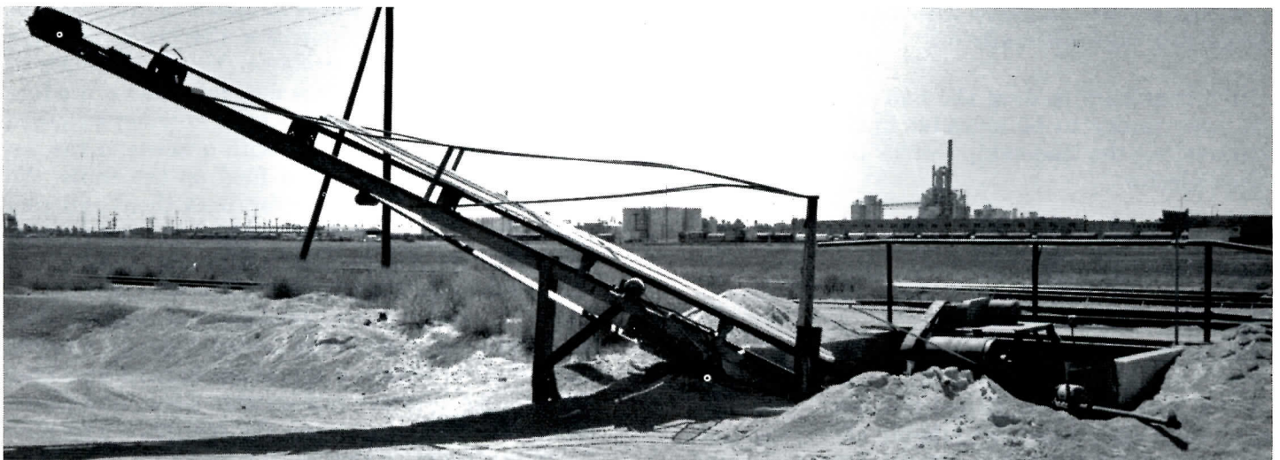
The elevator belt which loads the material into a waiting dump truck. Still more detail! The belt guard on the motor was wildly askew. The pipe in the lower right corner may part of a pumping system. It has a small motor attached to it which can be seen here and in the photo above. The industry in the background is Proctor and Gamble. Photo by Bob Werre
