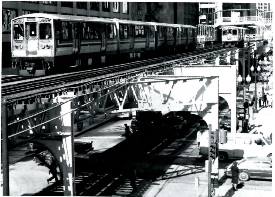
Elevated rapid transit trains in Chicago operate uninhibited over busy street traffic below.
