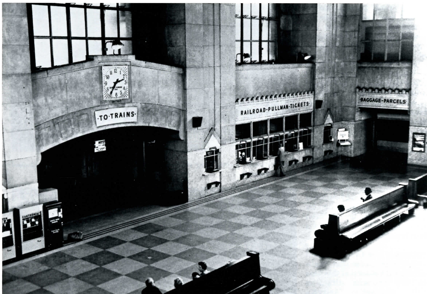
Part of the station's waiting room, 1957.
