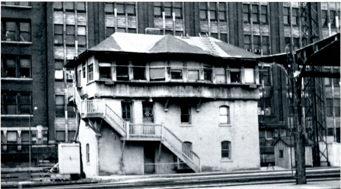
Polk Street Tower controlled NYC, RI, and NKP trains at Chicago’s LaSalle Street Station.
