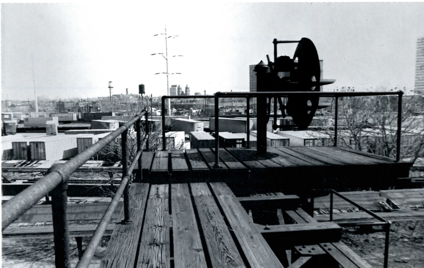
View showing top of PRR signal structure at Englewood (Chicago) Illinois. Note the wood footwalk planking.
