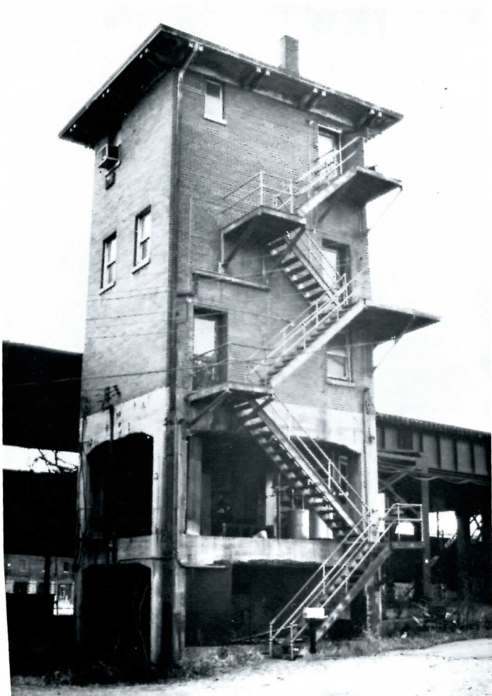
This 5-story interlocking tower serves the former C&O/ L&N elevated mainline near downtown Cincinnati.
