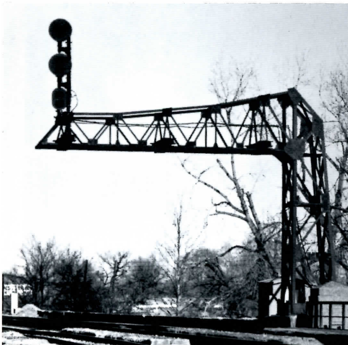
NYCRR cantilever signal structure at South Bend, Indiana.
