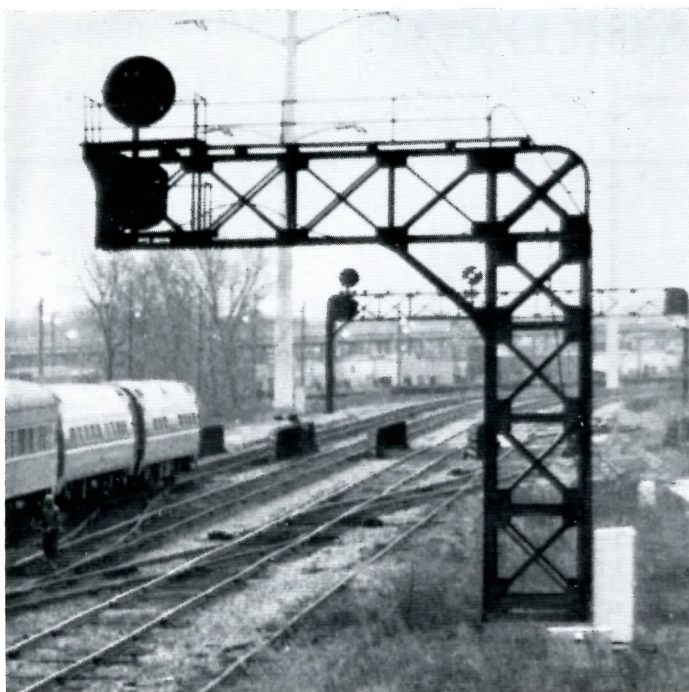
PRR cantilever tower at Englewood (Chicago) Illinois.
