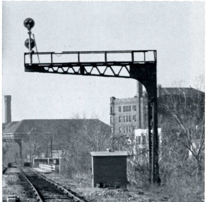
Rock Island structure at 65th Street in Chicago, Illinois.
