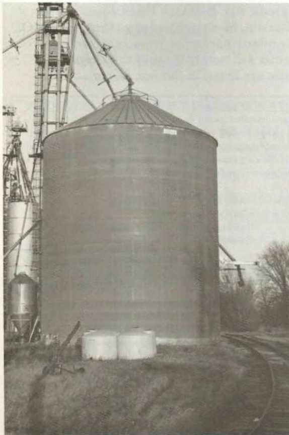
New Badgerland Coop grain storage silos. Ertl storage bins could make a good starting point for this industry.
