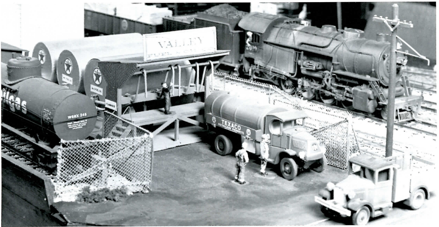
A scene at Valley Fuel and Oil Company's truck loading facility. A Reading I-10SA can be seen drifting by with a freight drag in tow.
