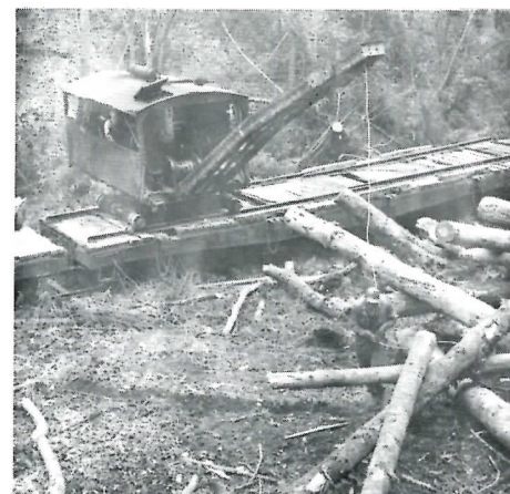
1903 American log loader at work along Lilly Fork.
