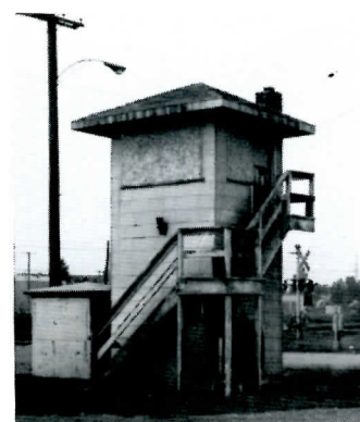
Abandoned grade crossing tower on Fort Street in Detroit. Now gone. Photo by Dave Held
