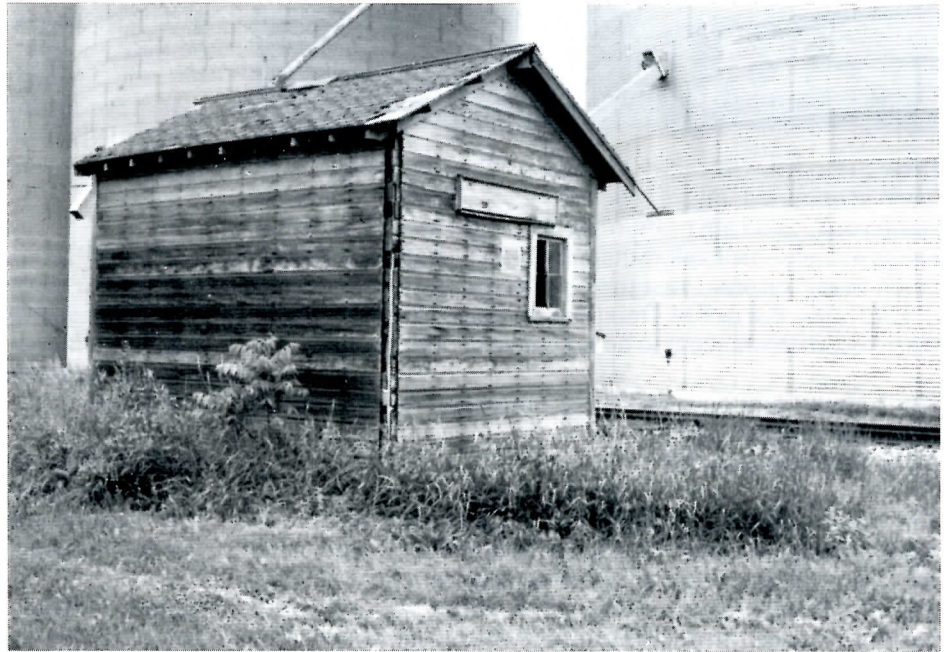
Rear view of Austinville depot. Note offset window on this side. Board spacing is about 5 inches. Photo by Bob Nicholson
