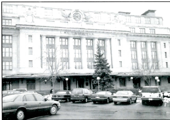
This is the street side of the Radisson Lackawanna Station Hotel in downtown Scranton. Steamtown is just on the other side, and a big indoor mall is just to the right of the photo.
