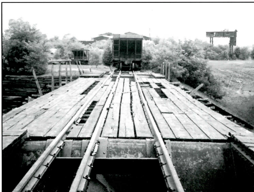
A top view of the coal trestle in Mt. Union with the transfer crane far in the background. These photos were taken in 1968.
