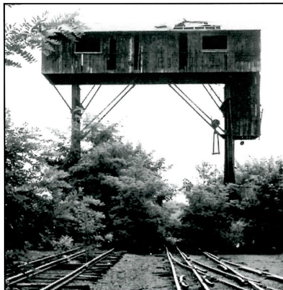
The transfer crane is a must if you model Mt. Union yard. It's where standard gauge cars received narrow gauge trucks.
