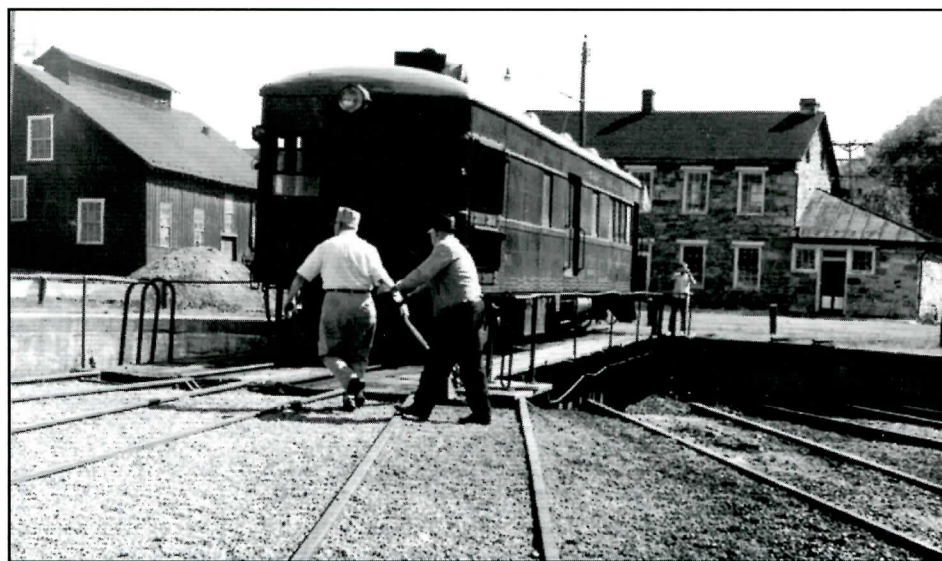
MI motorcar, which I nicknamed the "Ruptured Duck" because of it's off key horn, rides the "armstrong" turntable at Rockhill Furnace. Note stone-farmhouse in background which became shop super's office.
