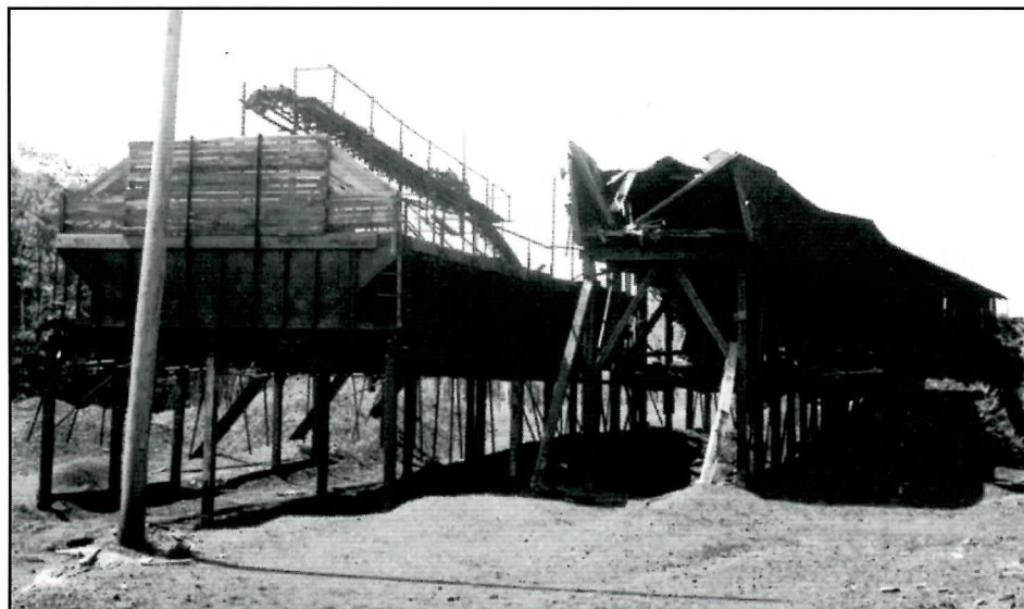
Above - Mine tipple around Alvan in the 1970s. Note hoppers used for loader at far right. Below - is a view from the opposite end showing the hoppers to the left. Photos this page Jeff Madden
