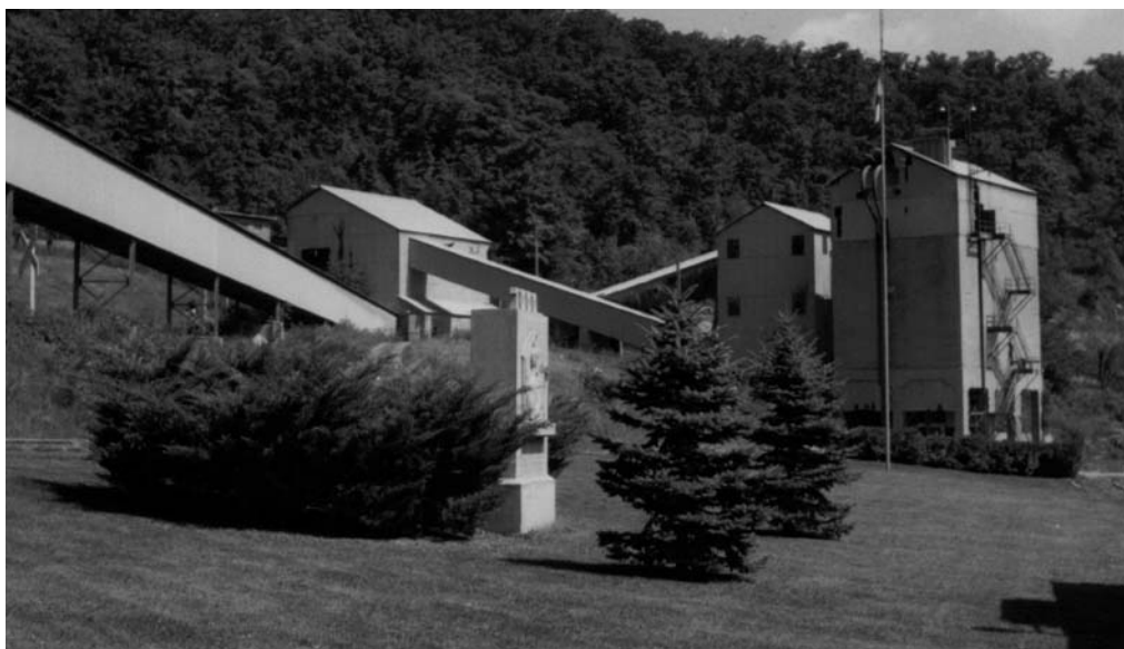
The processing complex where the limestone is crushed and processed. The covered conveyers move the stone to different process.
