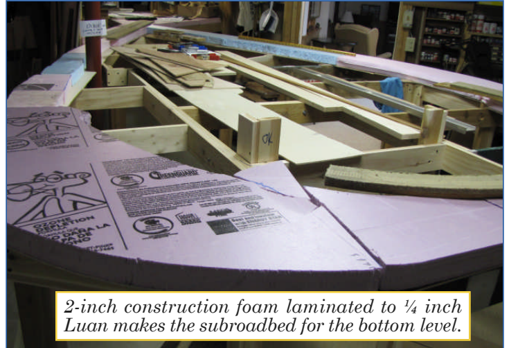
Above: Open grid benchwork for the new peninsula is up on L-shaped legs. The lower staging loops go on this.
