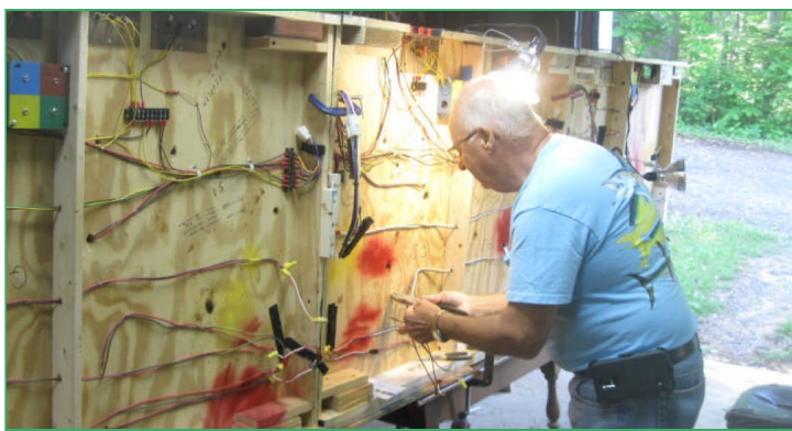
Doug Boomer preparing modules for upgrade.
