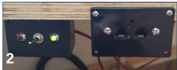
Above: Turnout panel and UTP panel
