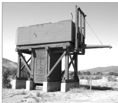
Arboles, Colorado. old D&RGW tender mounted and used as a water tank.
