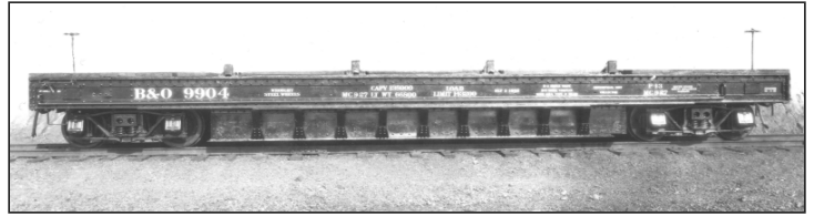
Number 9904 seen above in 1927 with no load, was the last of these class P-13 cars built for the B&O.
